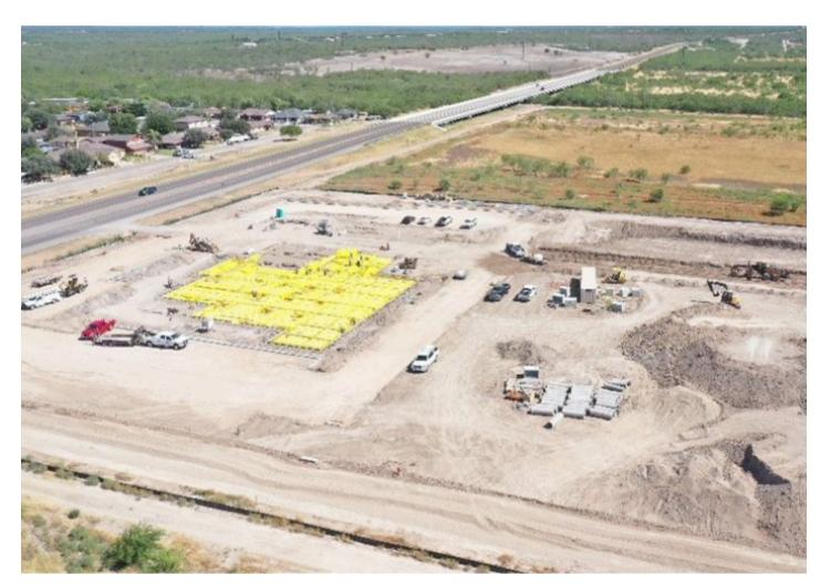
The NEW Public Safety Building for the City of Rio Grande City is progressing right on time! The underground maintenance has been completed and we are preparing to form and rebar the area in preparation to pour the foundation, as well as the curbing and framing of the parking lot. This new Public Safety Building will house our RGC Fire Department and RGC Police Department and we are excited for this project to be completed by Spring of 2024!
